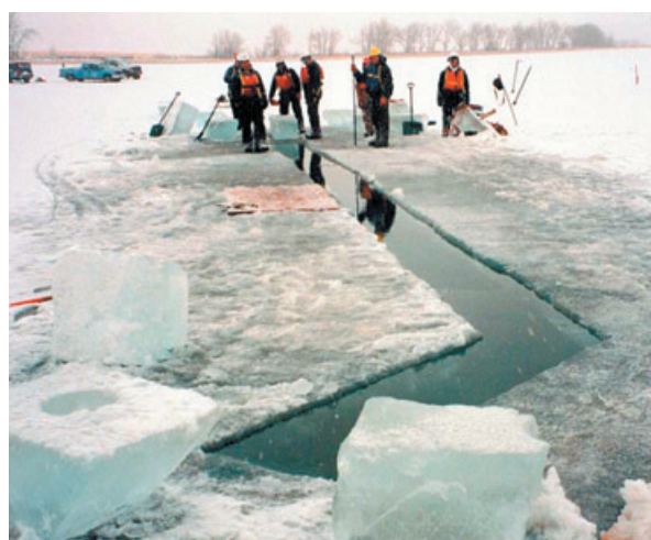
Below: a slot cut into ice allowing oil to rise and flow to a collection point.
