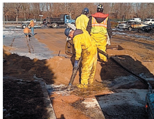
Workers recover sorbent material that has been used to clean an oiled road.
