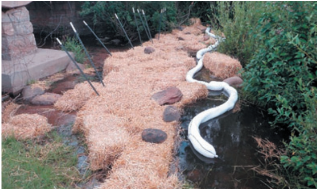
Above left: straw used to hold back and absorb low quantities of oil.
