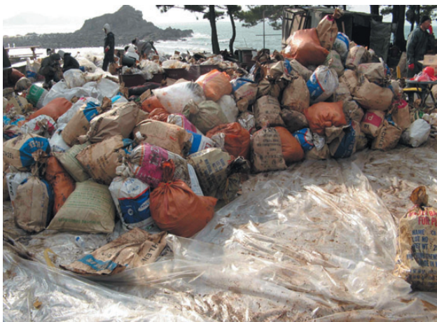
On-site, temporary storage of waste in sacks laid on impermeable sheeting at the beachhead.
