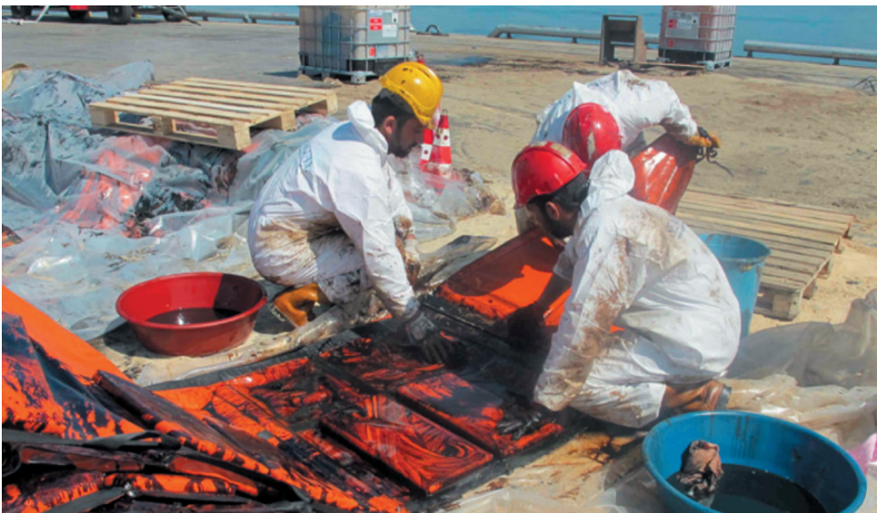
Washing containment boom prior to reuse.
