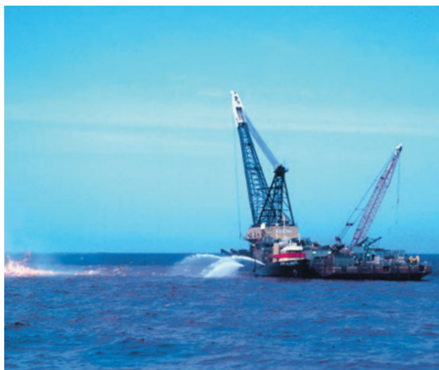
Some spills present specific safety risks.
